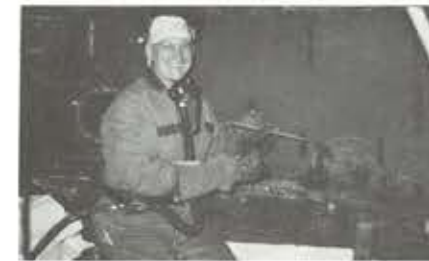
Welder Nick Foglietta, plying his trade on the floor of #8 Digester.
