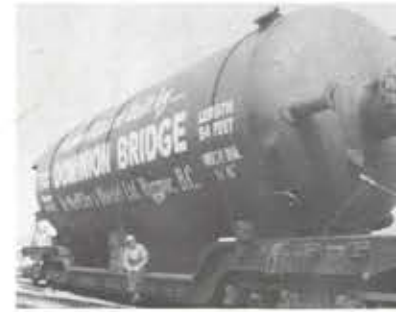
One of the digesters that the Harmac Railroad carried to the plant, back in 1948. That's brakeman Al MacPherson on the flat car.
